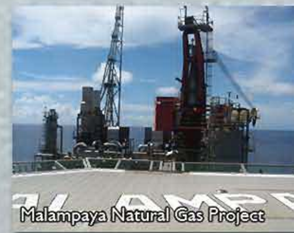
Malampaya Natural Gas Project
